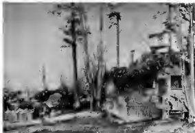
Figure 52. Another method of breaking identifying shadows is to attach silhouettes of plywood or other rigid materials to the walls.
